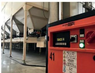
Fig. 2 – Aerotermino in reparto silos pastificio
